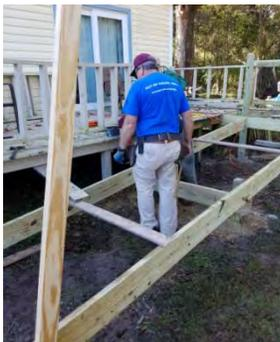
The team constructing the ramp removed the steps from the deck and then built a new 5'x6' deck to connect the ramp. The ramp would eventually be 28' long. The team dug holes for posts at prescribe locations, placed posts and filled holes with concrete. Decking, along with railings, was added to the ramp. They also replaced the old deck stairs at a rear entrance to the house.
