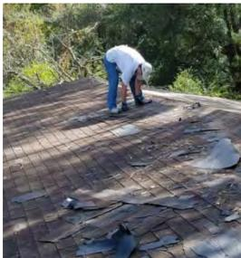
Monday thru Friday, the volunteers were broken up into two teams. One on roof repairs, the other on constructing a deck and ramp. The roof required much dismantling and the removal of the old shingles, various pieces of roof sheathing and fascia. Many of the rafters also needed repairs. The team worked hard and finished the roof on Friday morning.
