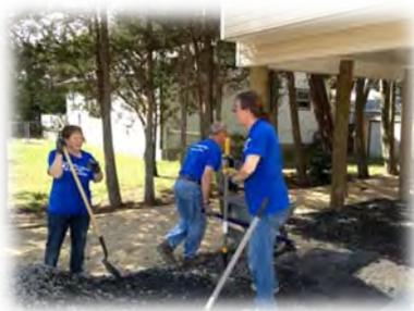
A team was dispatched to Tuckerton, NJ to spread 20 tons of crushed stone under a rebuilt elevated home also close to completion. With only two wheel barrows and mostly senior citizen workers, this was completed in one day.
